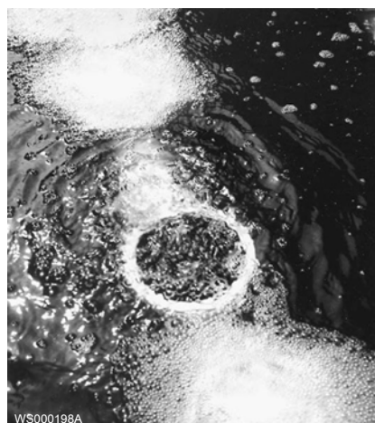
Figure 28: Excessive air discharge
